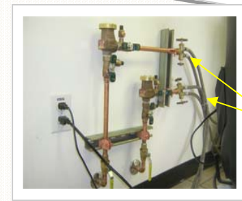
Typical PVB Installation
